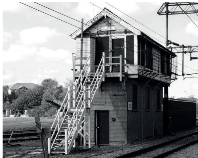
SIGNAL TOWER AT BISHOP'S STORTFORD TRAIN STATION
