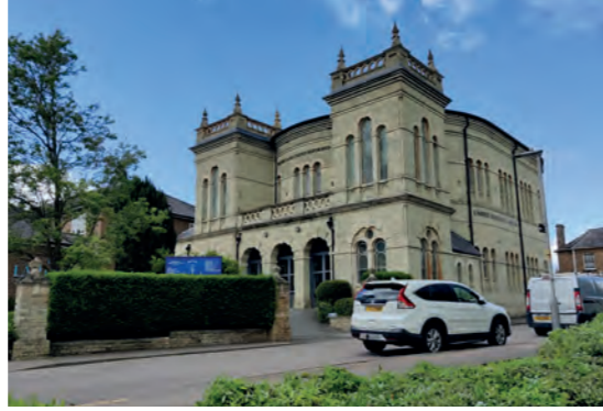
⑨ Water Lane United Reformed Church
