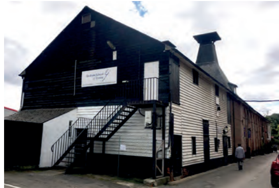
⑦ Former South Street Maltings
