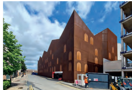
20 Multi-storey Car Park 1
